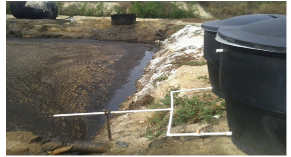
Dual tank setup (2000L combined capacity) drip dosing (gravity) through PVC tubing and spherical valves
