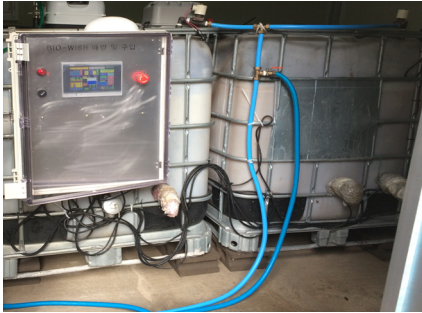
Dual IBC tote system (2000L combined capacity) dosing BiOWiSH™ Aqua into municipal STP raw inflow through a metering pump controlled by local PLC
