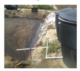
**Liquid Dosing:** Dissolve the BiOWiSH<sup>™</sup> powder concentrate in clean water (at a minimum rate of 10 L/kg). Active solution can be drip-dosed directly to the lagoon inflow or for lagoons with HRT > 24 hours, poured into the lagoon on a weekly basis.
