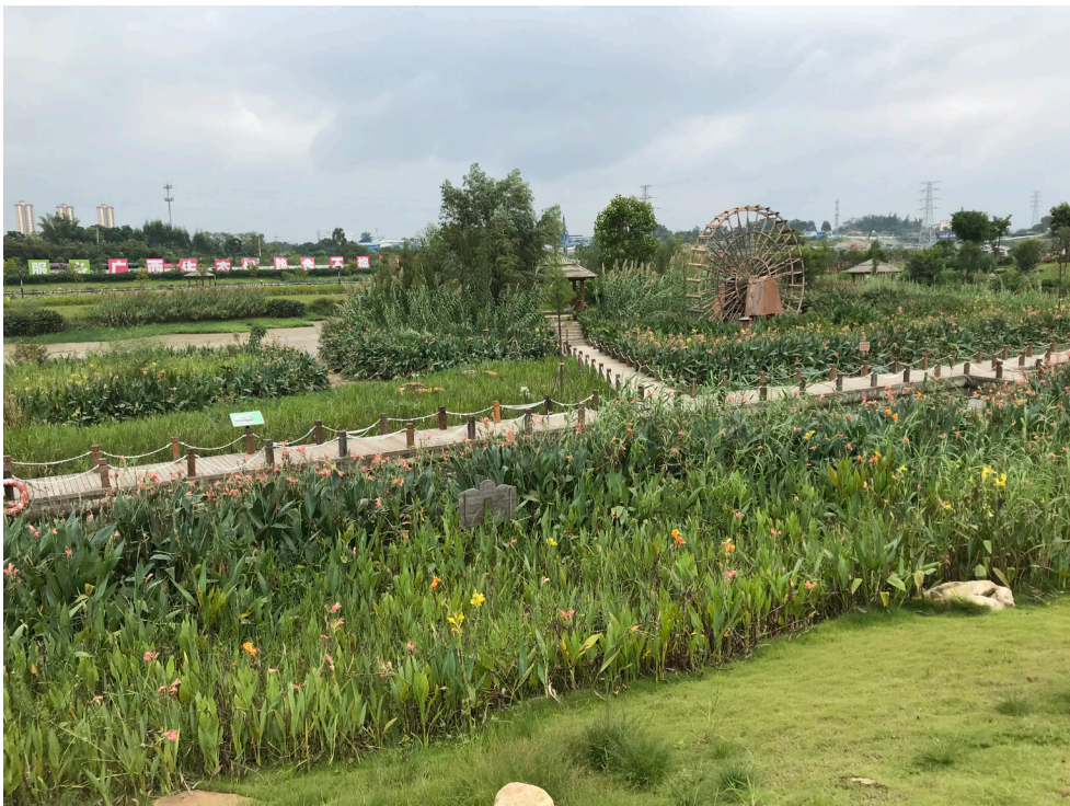
Figure 3: Surface Flow Wetland in Nanning, China
