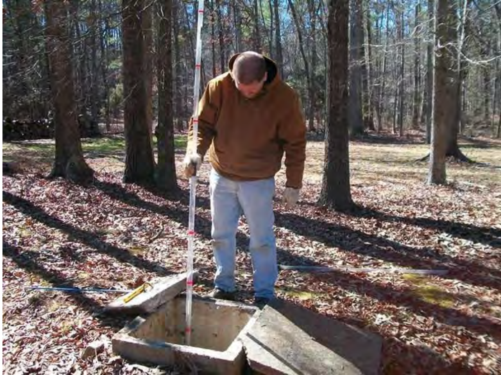
Measuring Solids Levels and Scum Layer Levels
