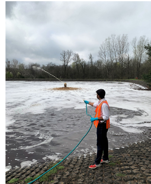
Dosing 1,000,000 leachate lagoon
