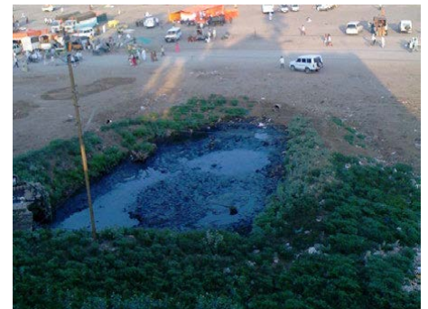
Dosing Station 3: Open Sewage Ditch
