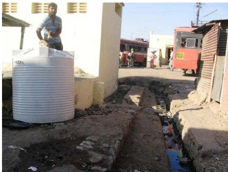
Dosing Station 1: Canal Opening
