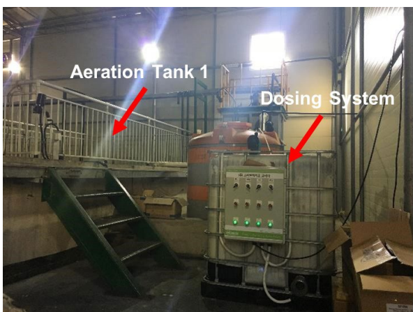
Fig. 3. 1000 Liter Tote for Dosing BiOWiSH®
