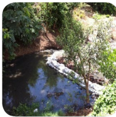
Figure 3. Sand bag location
