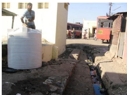
Dosing Station 1: Canal Opening
