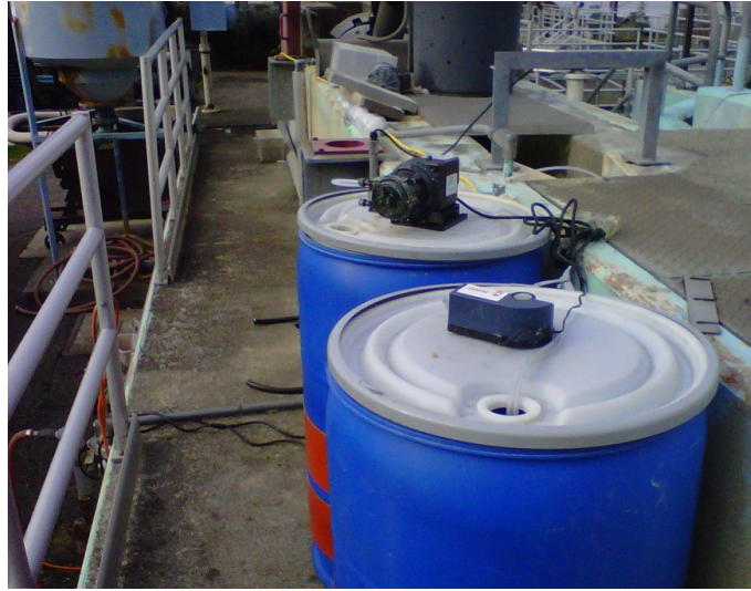
Figure 5 - BiOWiSH™ Dosing Set Up
