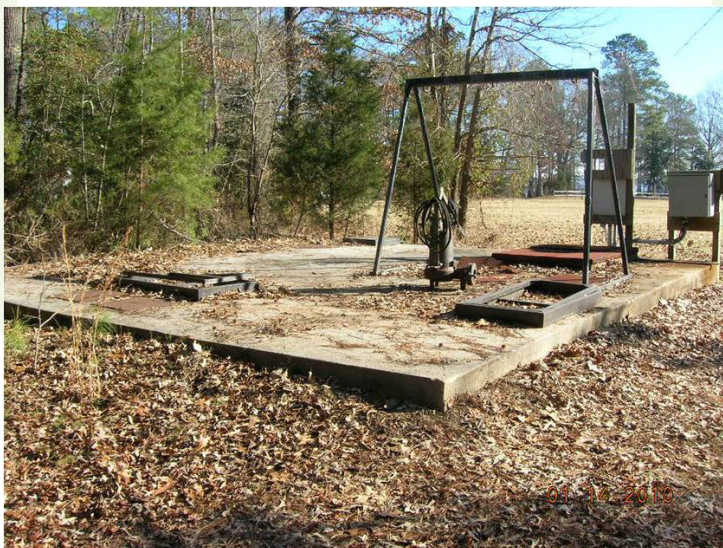
E Section Tank cluster - 113,000L sludge tank, 18,000L central tank and 56,000L effluent tank in series - discharging to a leach field in the background
