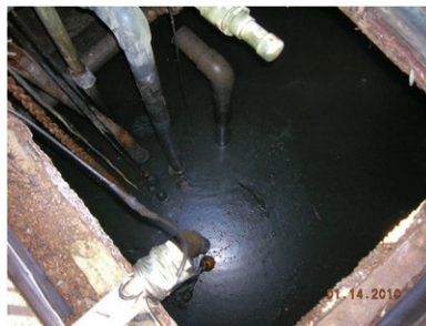
View inside the effluent tank
