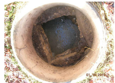
View inside the cover of B section bathroom tank
