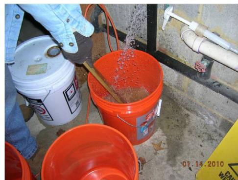
Pre-batching tank doses in 5-gallon buckets
