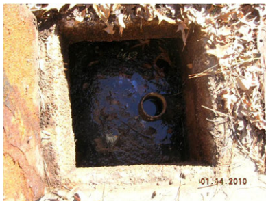
View inside sludge tank cover
