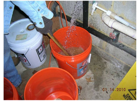
Pre-batching tank doses in 5 gal buckets
