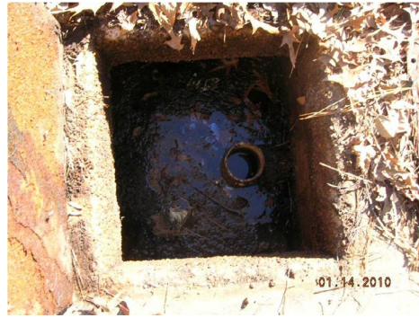
View inside cover of B section bathroom tank
