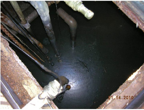
View inside effluent tank
