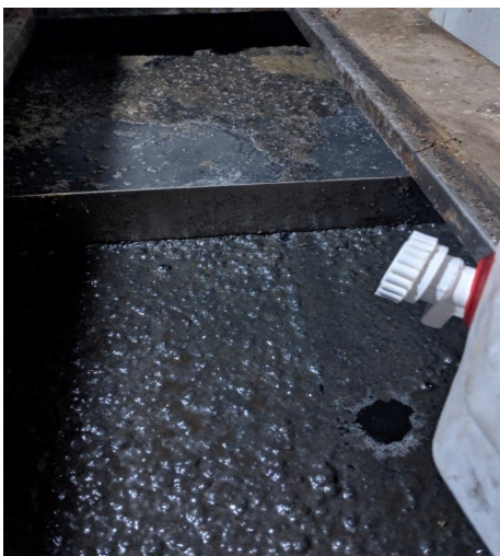
Continuous drip dose of BiOWiSH® Aqua FOG in grease trap
