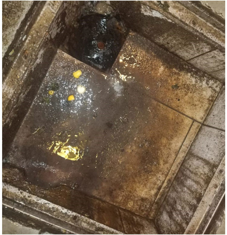
Clean drainpipe after 21 days of BiOWiSH® Aqua FOG treatment
