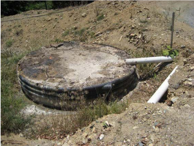
Tallow Dam Before
