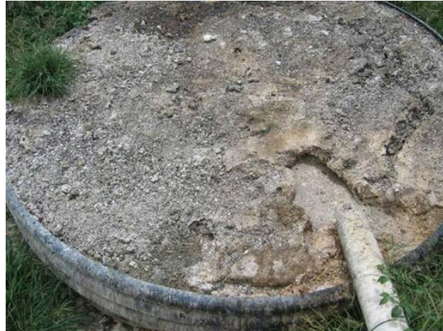
Tallow Dam After
