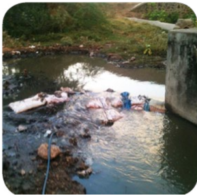
Figure 2: Initial dosing point
