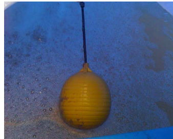
Float Valve Inside Dosing Tanks
