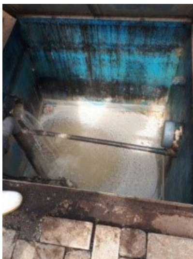
Figure 1: Effluent control tank 1
