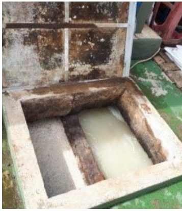
Figure 3: Effluent control tank 3
