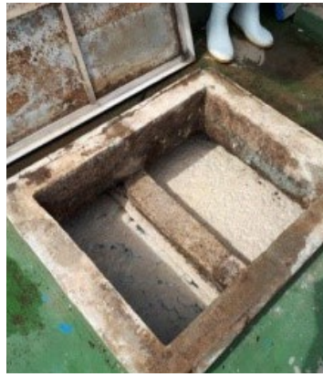
Figure 4: Effluent control tank 4
