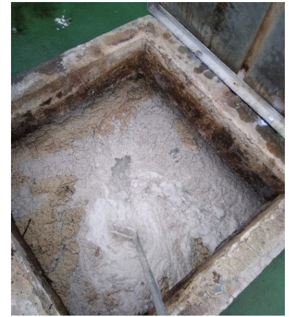
Figure 20: Sludge tank after BiOWiSH®
