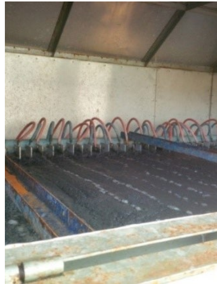
Figure 11: Electrocoagulation unit of the main treatment plant
