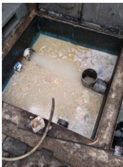
Figure 2: Effluent control tank 2
