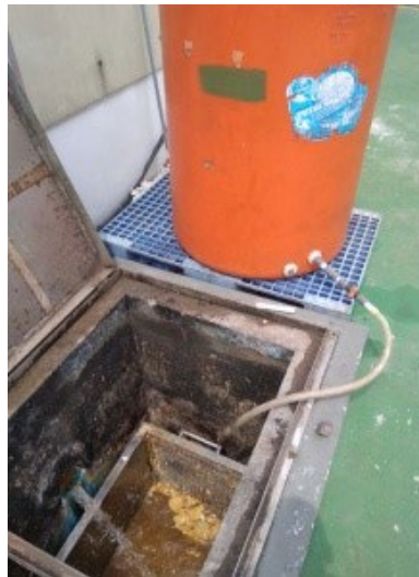
Figures 6, 7, & 8: Grease trap in the food seasoning treatment process
