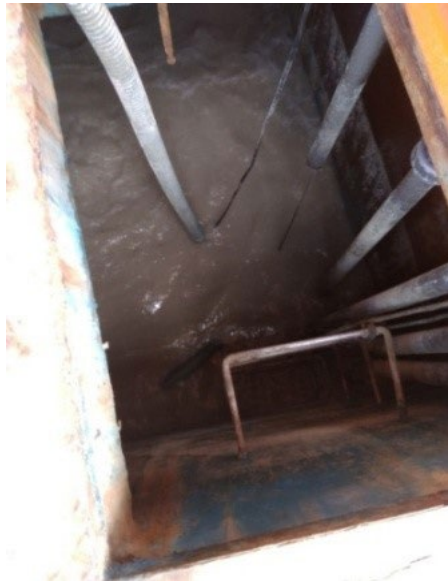
Figure 10: EQ Tank of the main treatment plant
