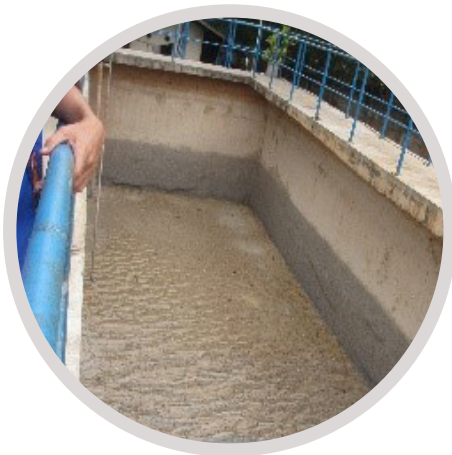
Sludge Holding Tank
