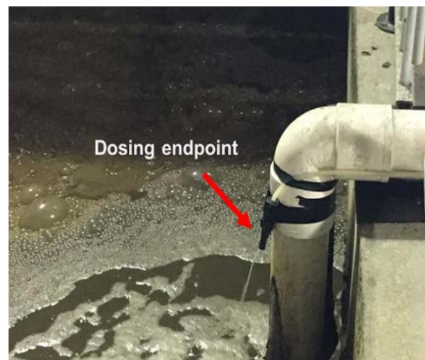
Fig. 4. Dosing Point in Aeration Tank 1
