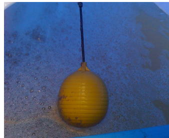
Float Valve Inside Dosing Tanks
